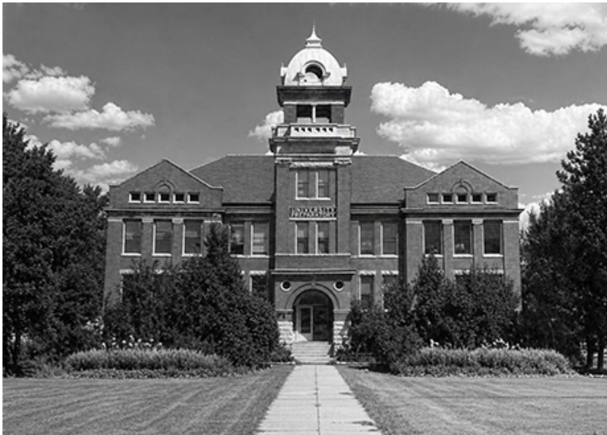
Central Hall -- The University Preparatory School
